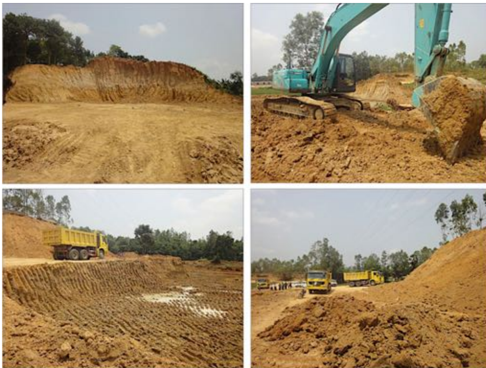
Fig. 5 Hill cutting soil is being transported as raw materials in the brickfields. Source: Department of Environment, Chittagong, 2014 and Ahmed, 2017
