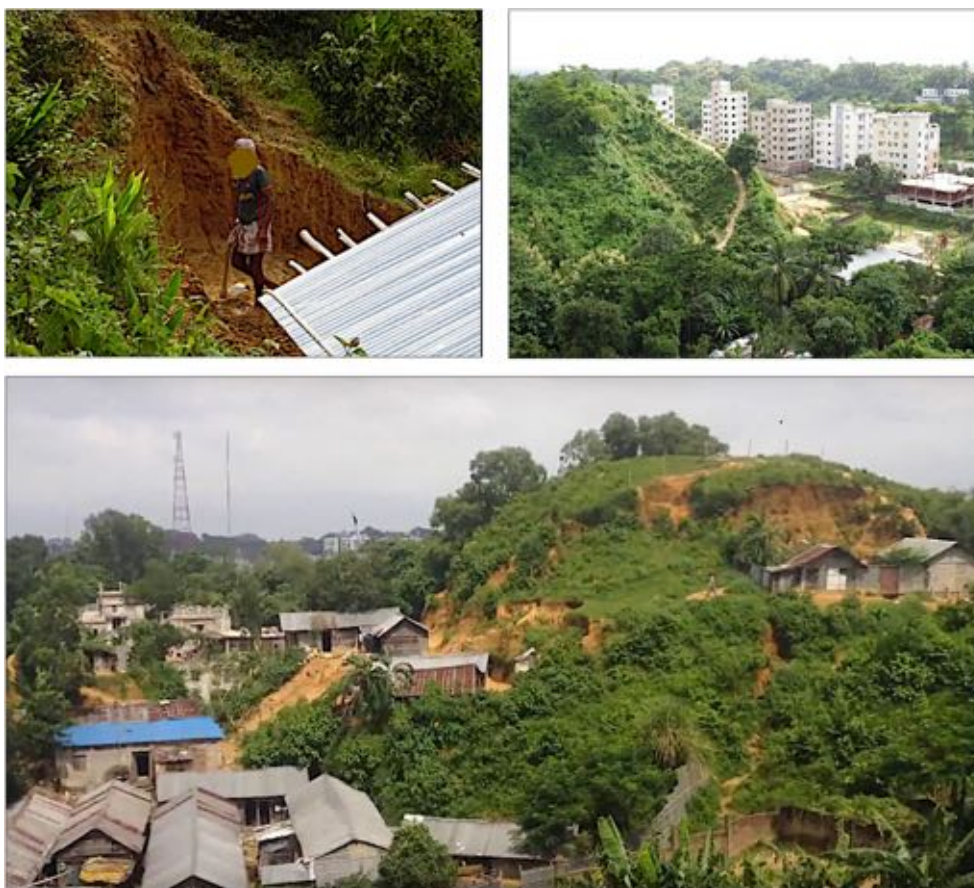
Fig. 6 Illegal hill cutting for development of residential housing in Chittagong City corporation area. Source: Bayes Ahmed, 2014 and Ahmed, 2017
