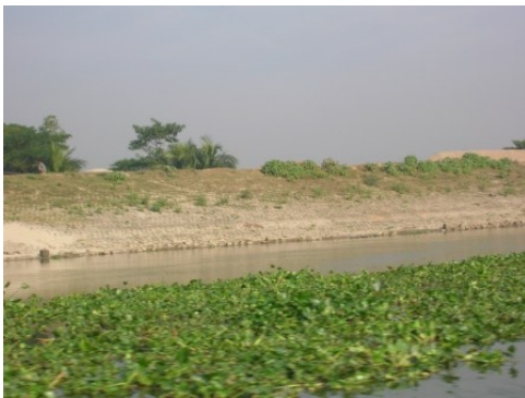
Figure 1: Meghna-Dhonagoda Embankment project
