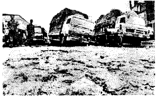
Fig. 1: Picture showing the damaged road condition with potholes.
