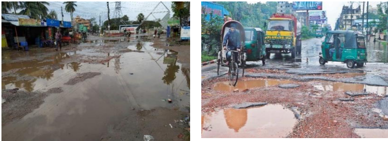
Figure 10 Damage of road due to waterlogging.
