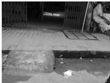
Figure 7: Improper kerb alongside the footpath.
